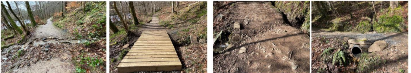
Before and after drain and boardwalk
