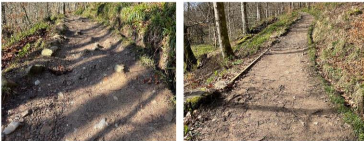
Before and after reduced trip hazards and revetment
