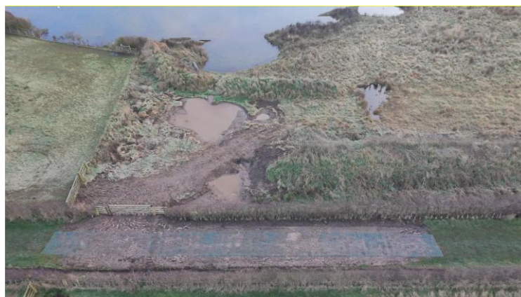
Aerial view of drained and resurfaced access (along bottom of photo), and of newly created ponds fed from culvert
