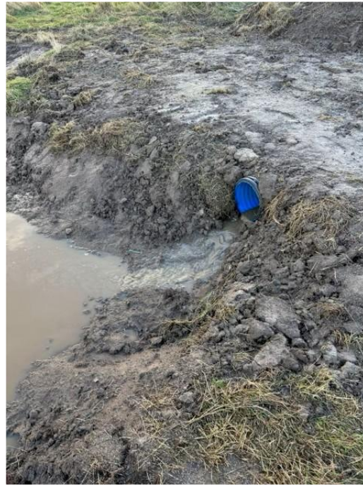
New culvert and drainage on wettest section of circular footpath
