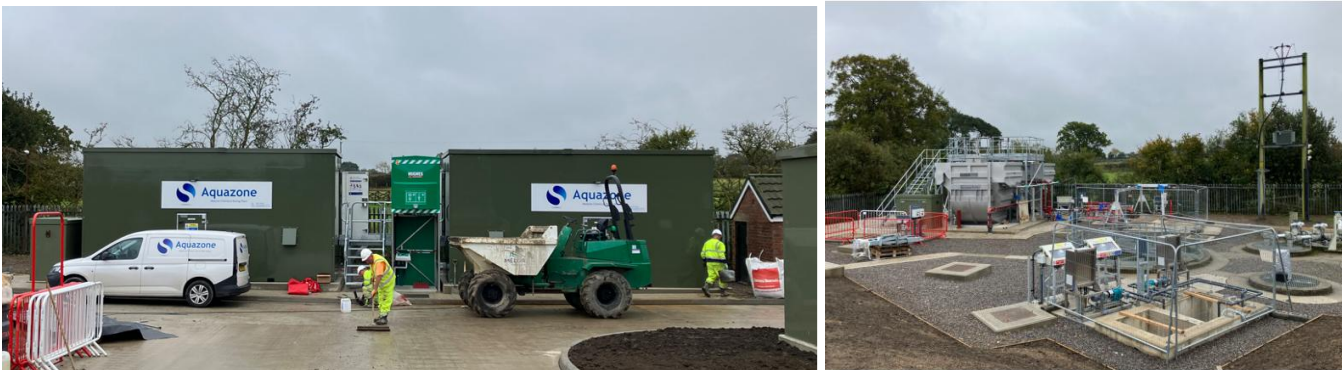
Chemical dosing kiosks (left) and mecana and secondary dosing cabinets (right) at New Moors STW
