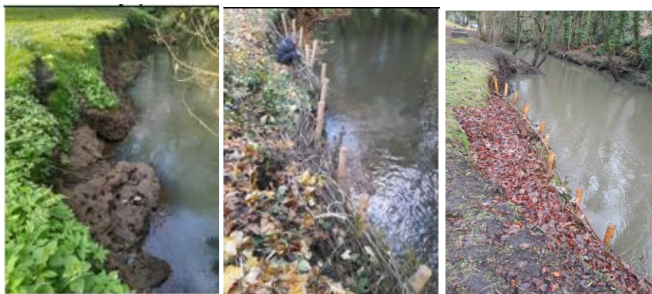
Eroded river bank in cemetery before (left), during (centre) and three months after (right) bankside repairs
