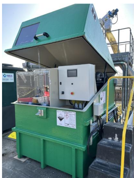
Chemical dosing kiosk containing storage tank and dosing pumps (left) and optimisation daily spot final effluent results (right) at Longhorsley STW
