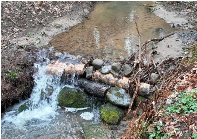
Woody dam with rapid sediment build-up from high flows, and a culvert being unblocked by volunteers
