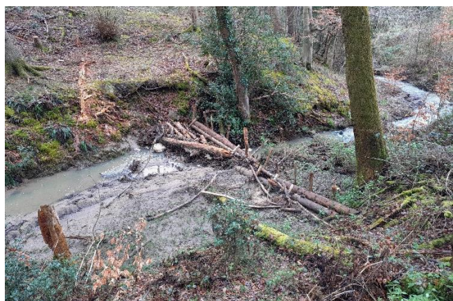
Woody dams installed upstream of culverts to protect them from debris
