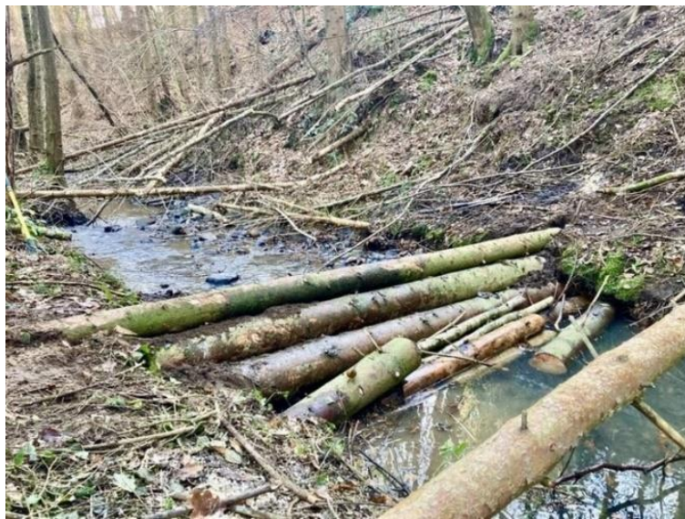
Woody dam construction
