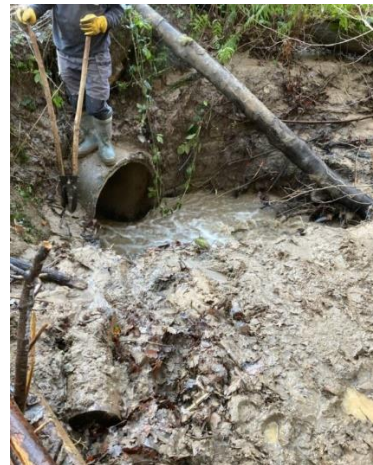
Woody dam with rapid sediment build-up from high flows, and a culvert being unblocked by volunteers
