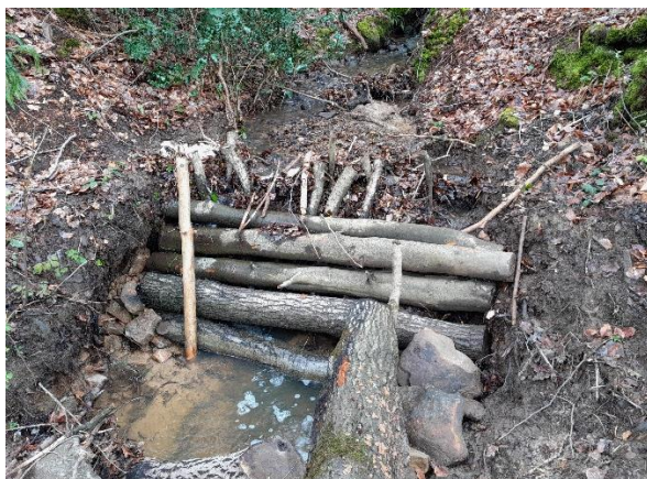
Woody dams installed upstream of culverts to protect them from debris
