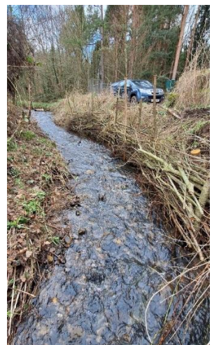
Willow barrier to prevent erosion
