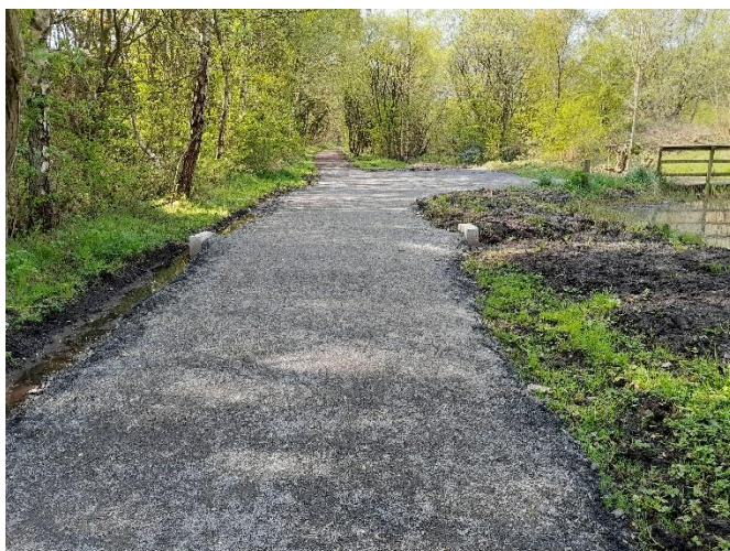
Path surfacing improvements with improved drainage
