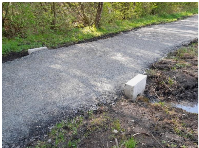
Better visual of wetland and meadow habitats from coppicing / culvert installation across newly surfaced path
