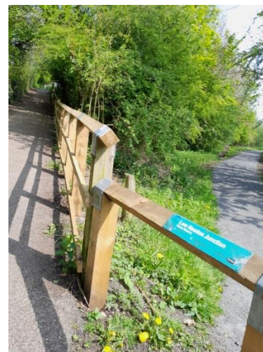
New fencing at the entrance to the site
