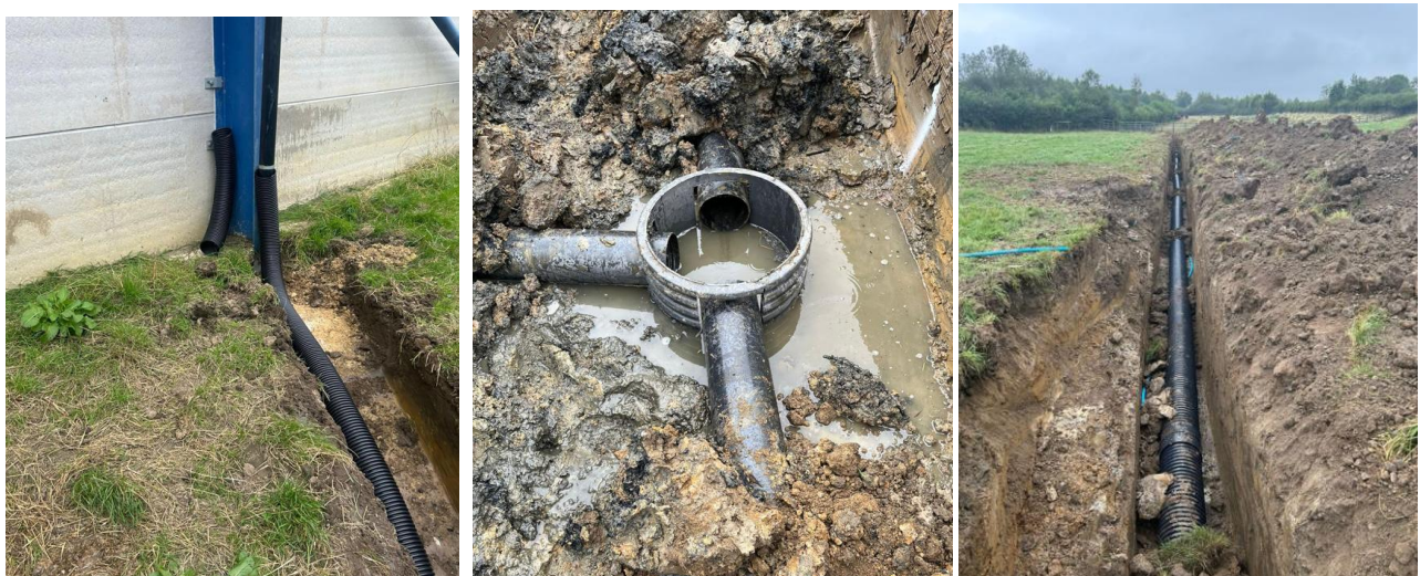
Capital works undertaken to trap and store clean rainwater, reducing run-off of dirty yard water and providing an additional source of clean water
