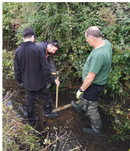
Staff and volunteers installing in-stream deflectors
