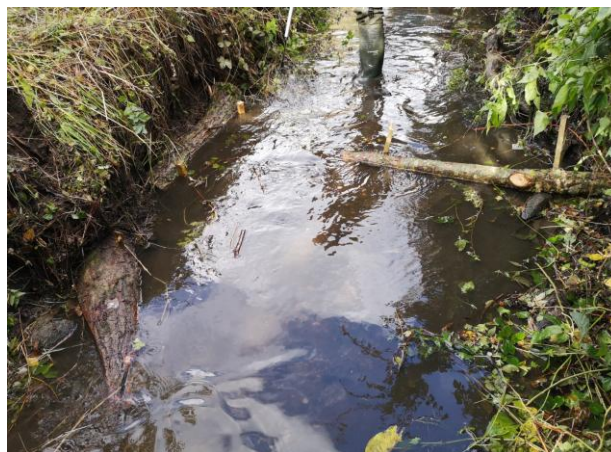
Completed deflectors in situ
