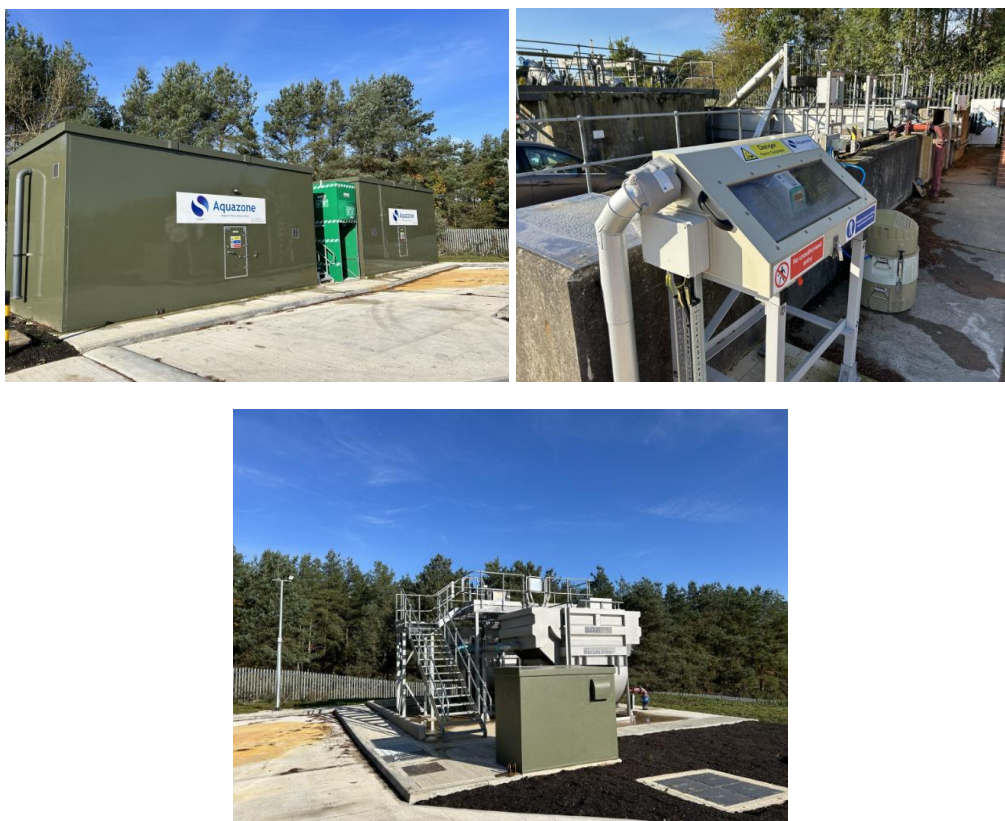
Chemical dosing kiosks and cabinets (top) and Mecana for tertiary solids removal (bottom) at Fishburn STW
