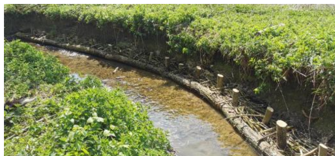
Willow spiling bank protection
