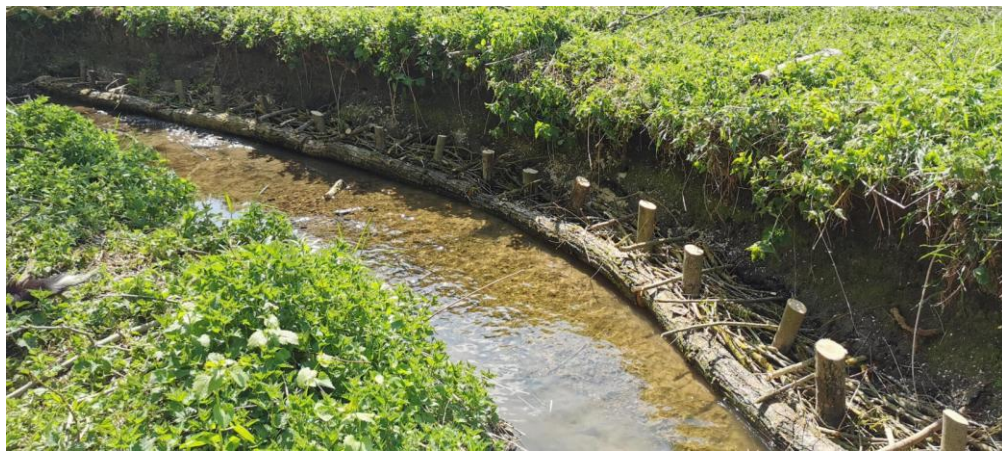
Installation of in-stream deflectors and bankside protection
