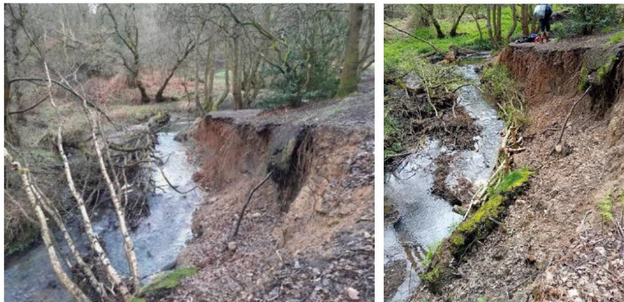
Before (left) and after (right) installation of bankside protection
