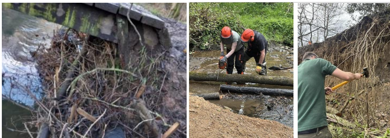
Bankside improvements to prevent erosion of bridge supports (left) and installing bankside protection
