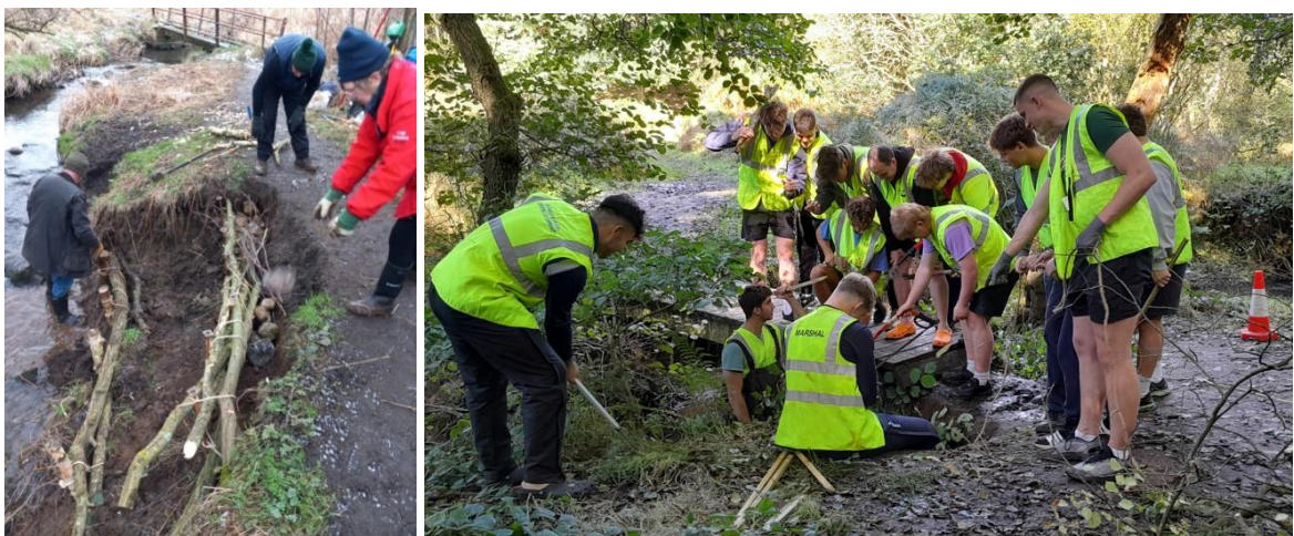
Volunteers assisting with bankside green engineering improvements
