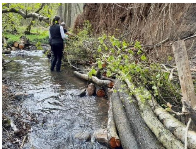
Bankside improvement reducing erosion
