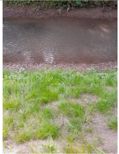
Embankment matting installed in Billingham Beck Country Park along watercourses, with newly establishing vegetation preventing erosion
