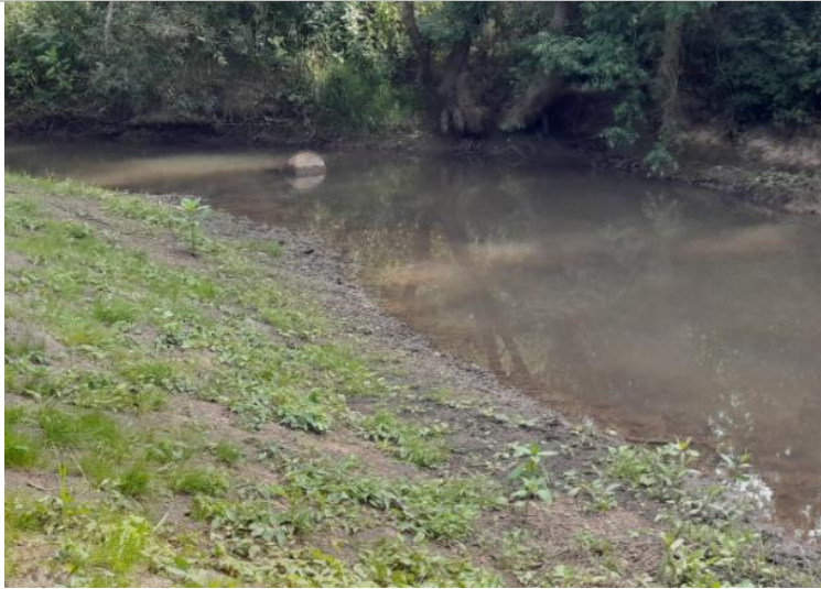
Embankment matting installed in Billingham Beck Country Park along watercourses, with newly establishing vegetation preventing erosion
