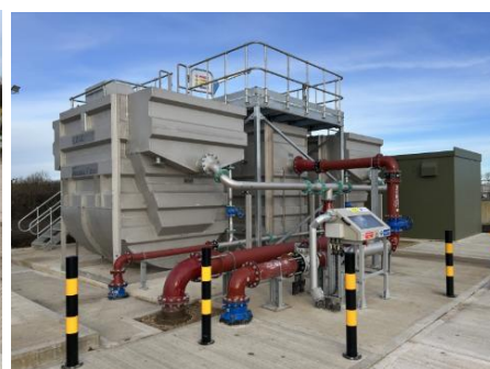
Sedgefield STW chemical dosing equipment and mecana (tertiary solids removal)
