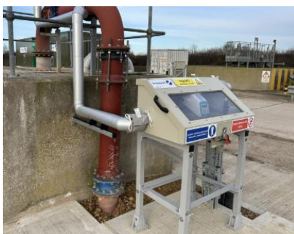
Sedgefield STW chemical dosing equipment and mecana (tertiary solids removal)
