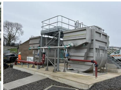
Carlton & Redmarshall STW chemical dosing equipment and mecana (tertiary solids removal)
