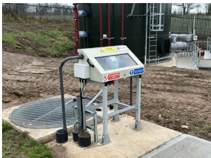
Carlton & Redmarshall STW chemical dosing equipment and mecana (tertiary solids removal)
