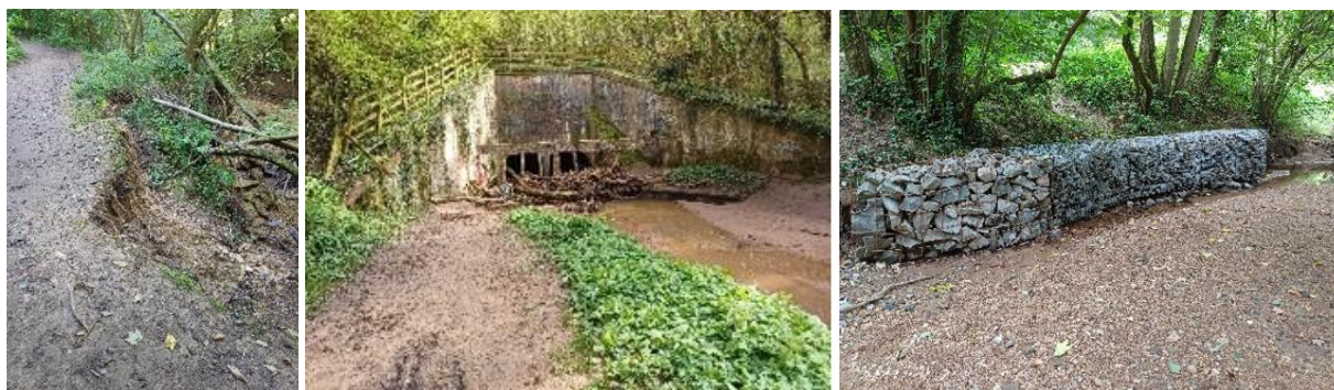
Using photos to monitor land-slip (left), monitoring dam build-up (centre), and gabion baskets for bankside protection (right)
