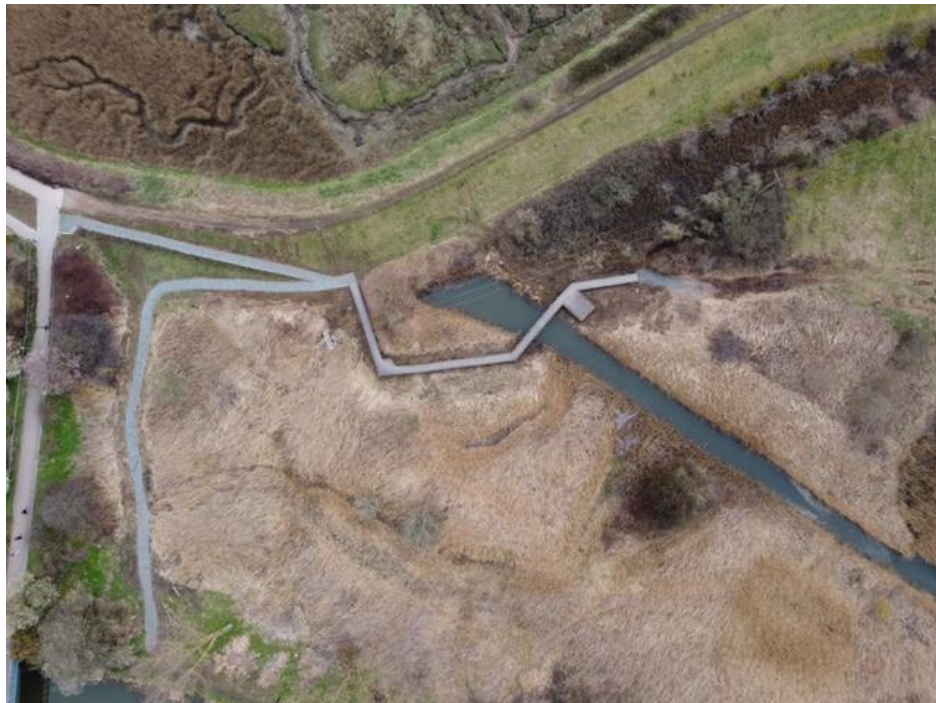
Aerial shot of the new footpaths, board walks and viewing platform
