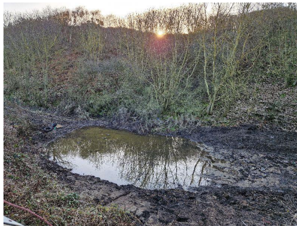
Newly excavated pond using mini digger
