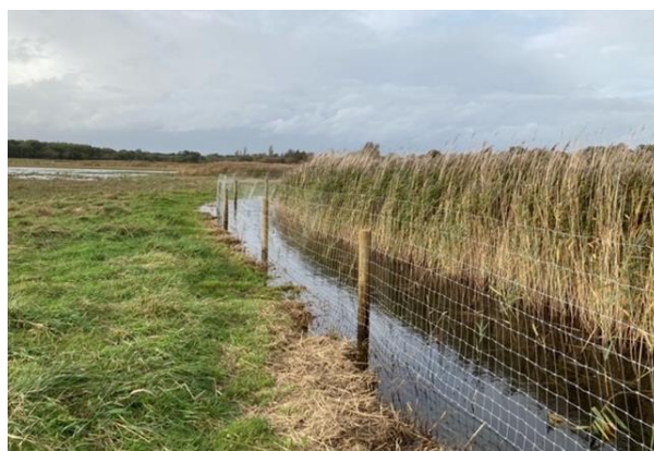
Anti-predator fence now in place, with in-ditch construction used where practicable
