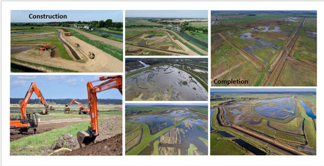
Figure 2: Creation of new wetland habitat at Carlton Marshes
