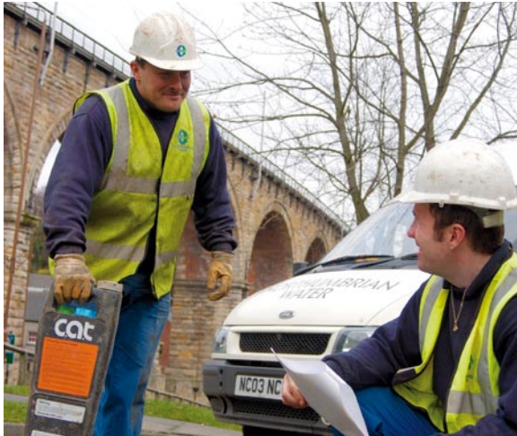
NWL's Alan Dixon and Mark McClean carrying out a mains repair.
