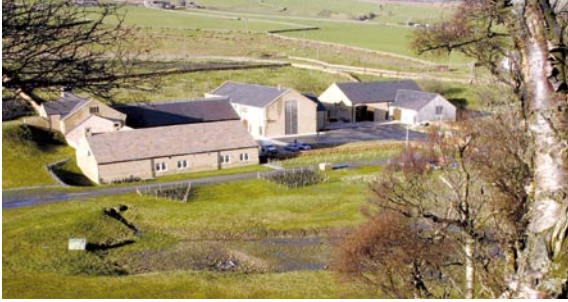
Wear Valley water treatment works in County Durham.
