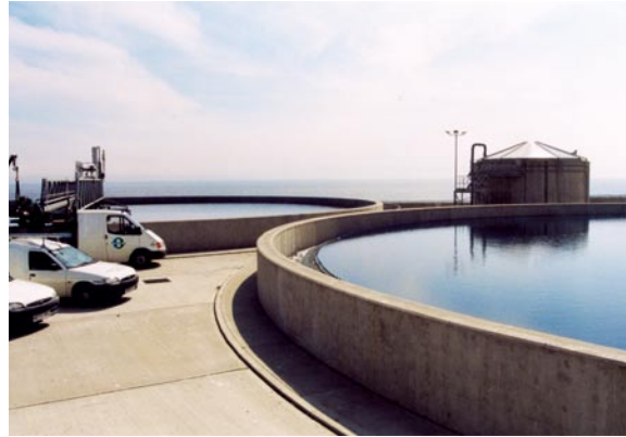
Hendon sewage treatment works in Sunderland.
