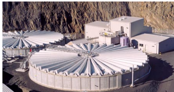
Inverclyde waste water treatment works, part of the Ayrshire consortium.
