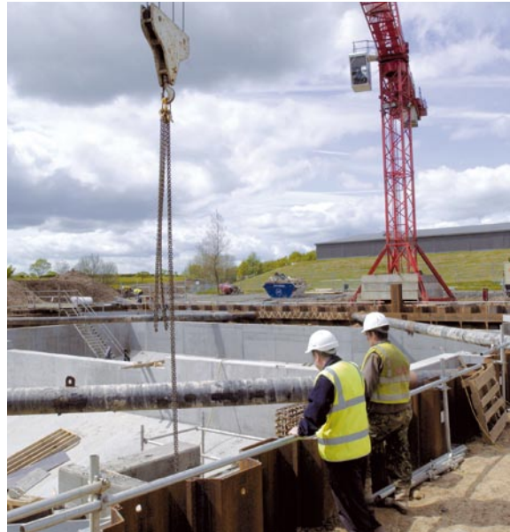
Construction work at Warkworth water treatment works in Northumberland.
