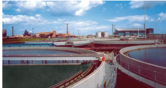
Bran Sands effluent treatment works in Teesside.
