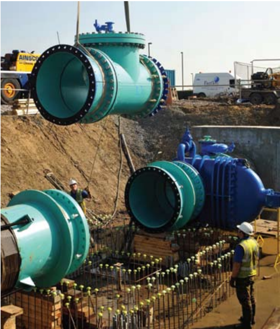
Mains cleaning programme – valve installation
