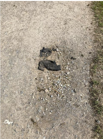
Path works before improvements: (Left) Typical pothole in footpath, showing wear beneath the membrane. (Right) Hump and incorrectly placed drain crossing the footpath
